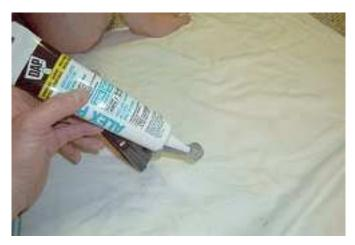
**Step 3** - To make installation easier, we recommend putting a dab of silicone on the face of the counter bored hole that the plastic washer sits into on the mirror stem. This will hold the washer in place during installation of all the other parts. Do this to both sides of the mirror post.
